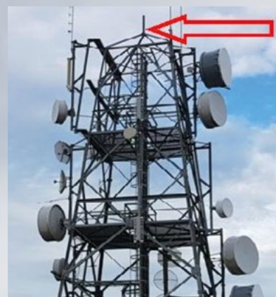
Figure 1: Top of a transmission tower that could be suitable as a survey reference object.
