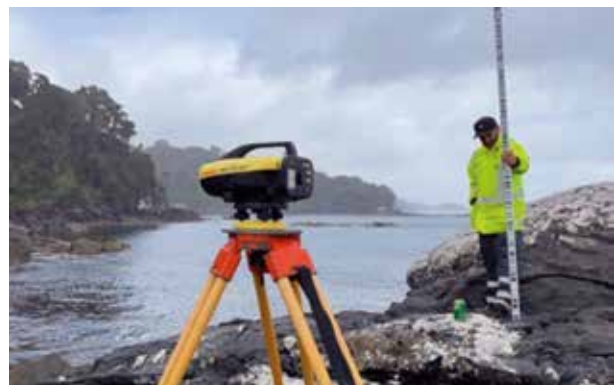
Establishing benchmarks near Christmas Village to establish survey control (Kate Downes, DML).
