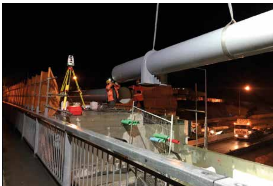
Nightworks – installation of the water main on Royal Road Bridge
