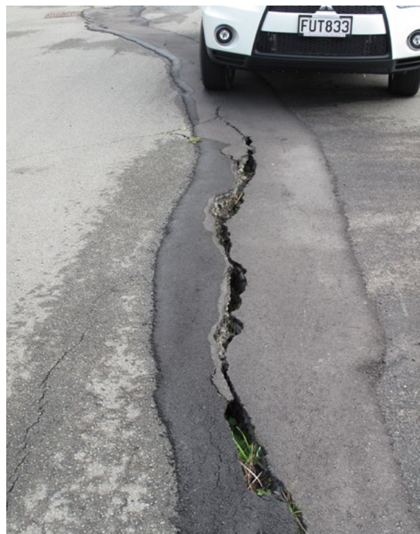
Earthquake damaged road, Redcliffe, Christchurch
