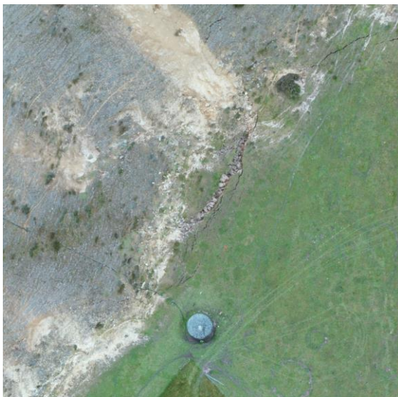
Fractures at the top of an escarpment
